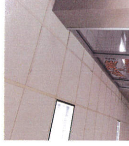
EXISTING HALL CEILING
